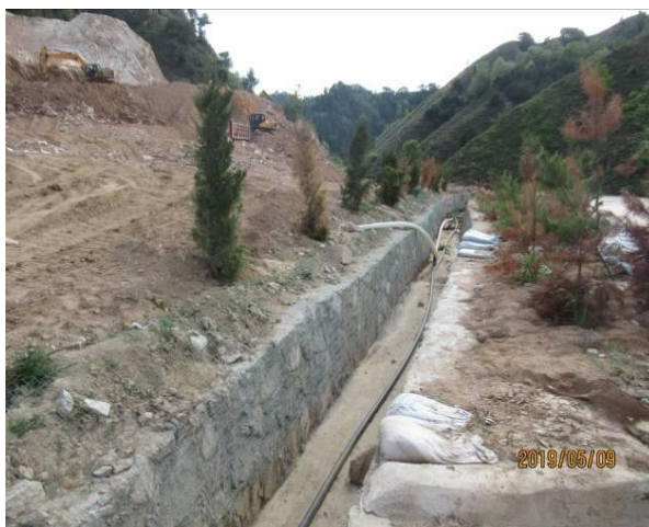
2-16 渣堆修建排水渠
